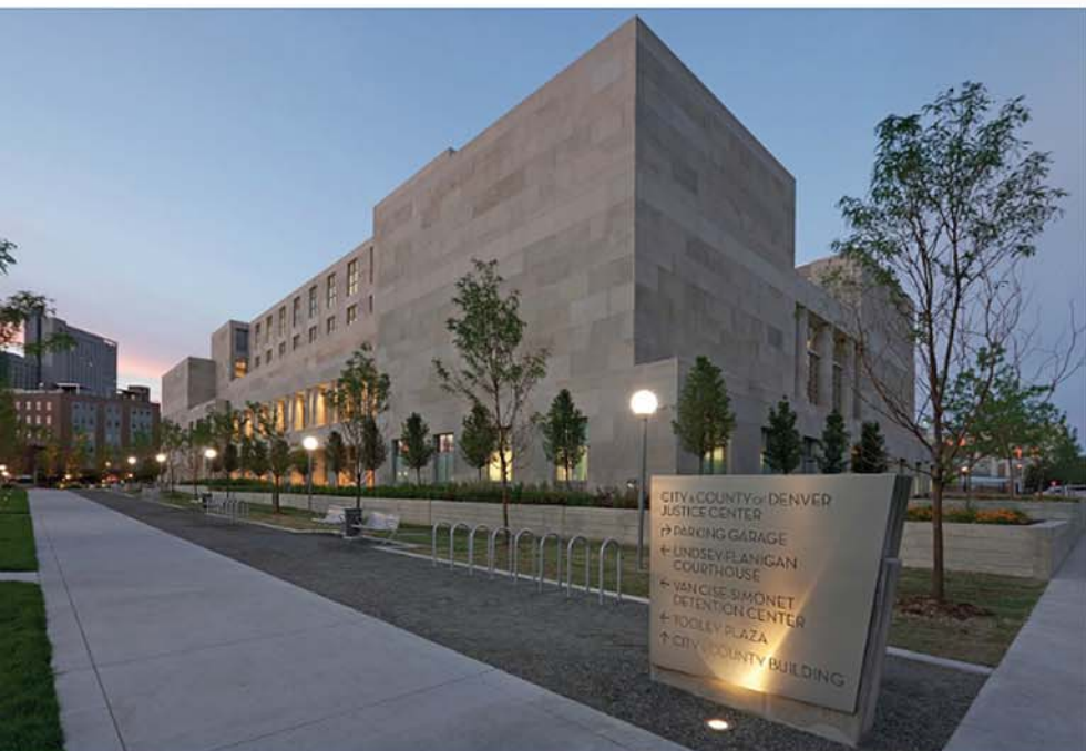
While the cost of the $160 million project was always kept in mind, it was important that the appropriate materials were used to blend the expensive building with its surrounding environment. "It is massive, so we tried to make it look more like a museum than a jail," said T. Lee Becker, FAIA of Herman-Cox Architects in Washington, DC, the lead design firm for the project. "That's why it is [comprised of] big shapes and covered in stone. We tried to design it as much as we could as a sculptural building." Photo by Frank Ooms Photography, www.frenkooms.com
