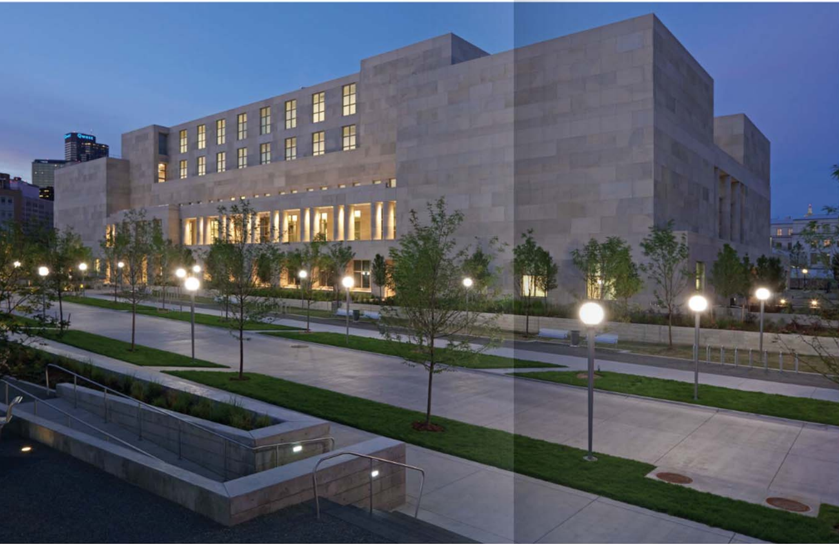
The exterior features 'shot sawed' Indiana variegated limestone with strips of Rustic Buff limestone. Photos on this spread and page 23 by Frank Ooms Photography, www.frankooms.com
