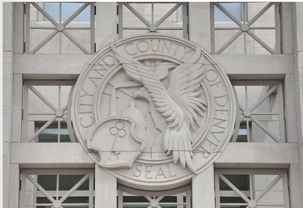
True craftsmanship is evident in the carving of the governmental seal of the City of Denver, which was placed over the entrance to the Van Cise-Simonet Detention Center. Bybee explained that this element consists of four panels that form an 8-foot-diameter circle. One carver completed the custom stone piece in five to six weeks. Photo by Henk Diepenbroek
