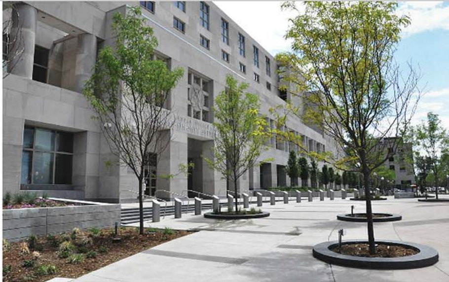
Portable jobsite cranes were used to set the variegated shot-sawed panels, which on average measured 8 feet, 5 inches x 4 feet, 5 inches. Photo by Hank Diepenbroek
